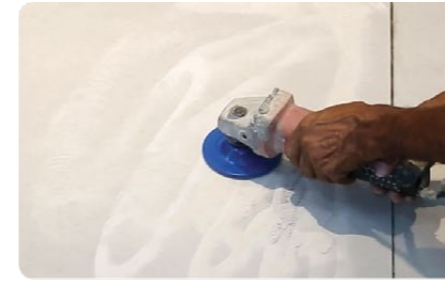
STEP 1 : GRINDING
